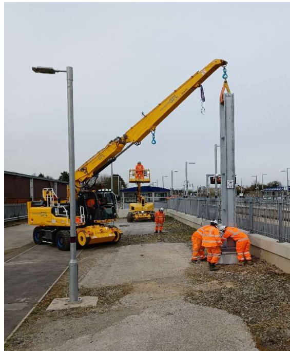
Easy does it: An overhead line mast is lowered into position behind Platform 1 on 15 th March 2022. Three were installed in not much more than an hour!
