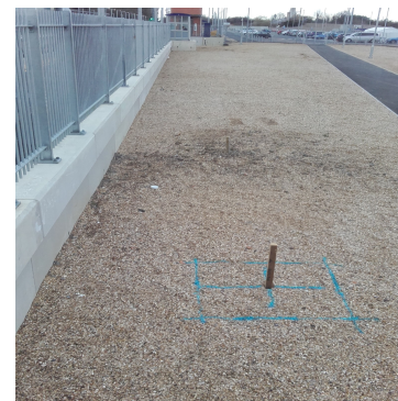
Pole position? Wooden peg behind Platform 2, marking where an electrification mast may be placed.
